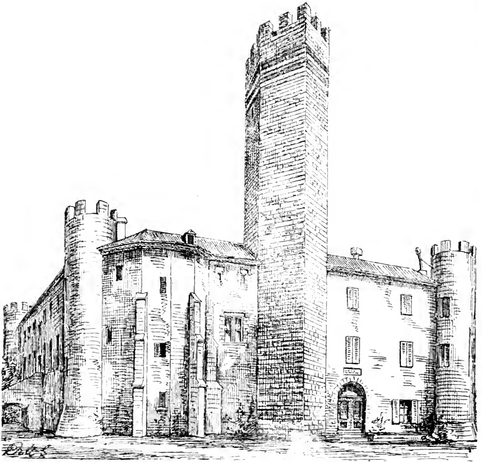
FIG. 212. CASTLE OF VILLENEUVE-LOUBET ( from the S.E. )
