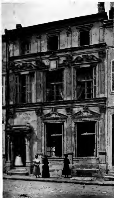
173. BAR-LE-DUC: HOUSE, PLACE ST PIERRE.
