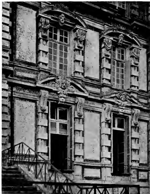
221. CHATEAU OF BEAUMESNIL: DETAIL OF WINDOWS.
