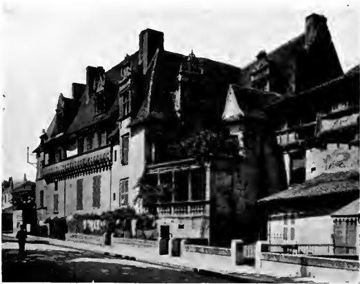
4. PERIGUEUX : HOUSES ON THE QUAY.
