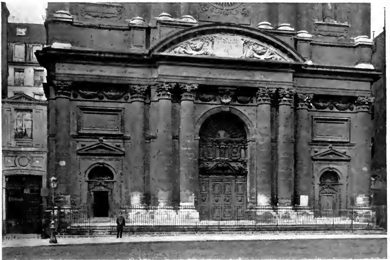
259. ST PAUL AND ST LOUIS: LOWER PART OF FAÇADE.
