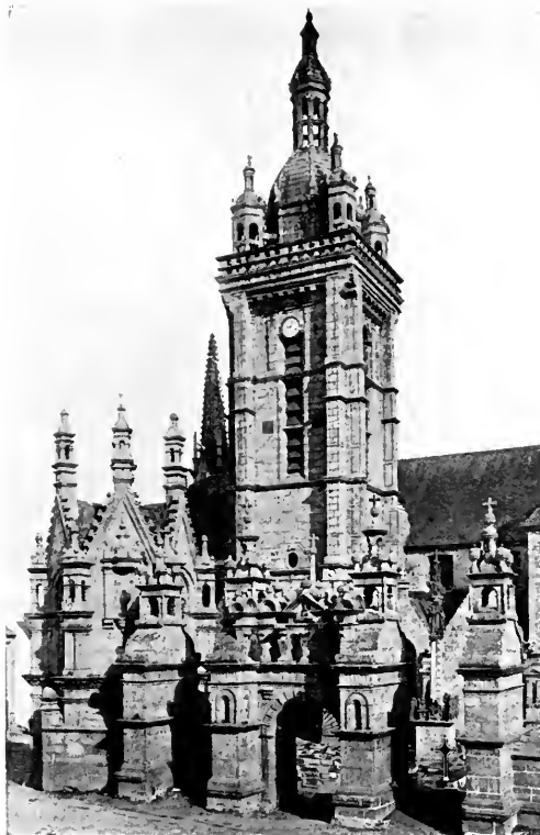
183. ST THEGONNEC: CHURCH AND CHURCH- YARD GATEWAY.
