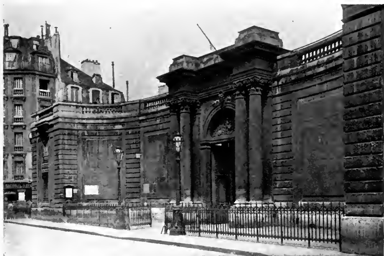
318. PARIS: HOTEL DE SOUBISE (NOW "ARCHIVES NATIONALES"), BY P. DE LA MAIRE (1706). ENTRANCE.
