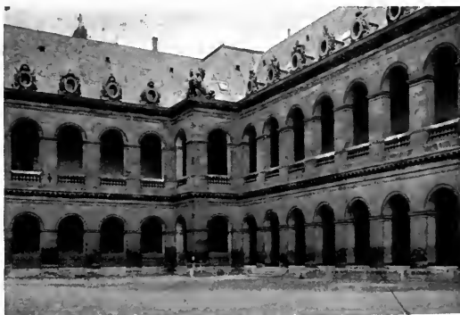
313. PARIS: HOSPICE DES INVALIDES, BY LIBERAL BRUAND (1671-74). PRINCIPAL COURT.
