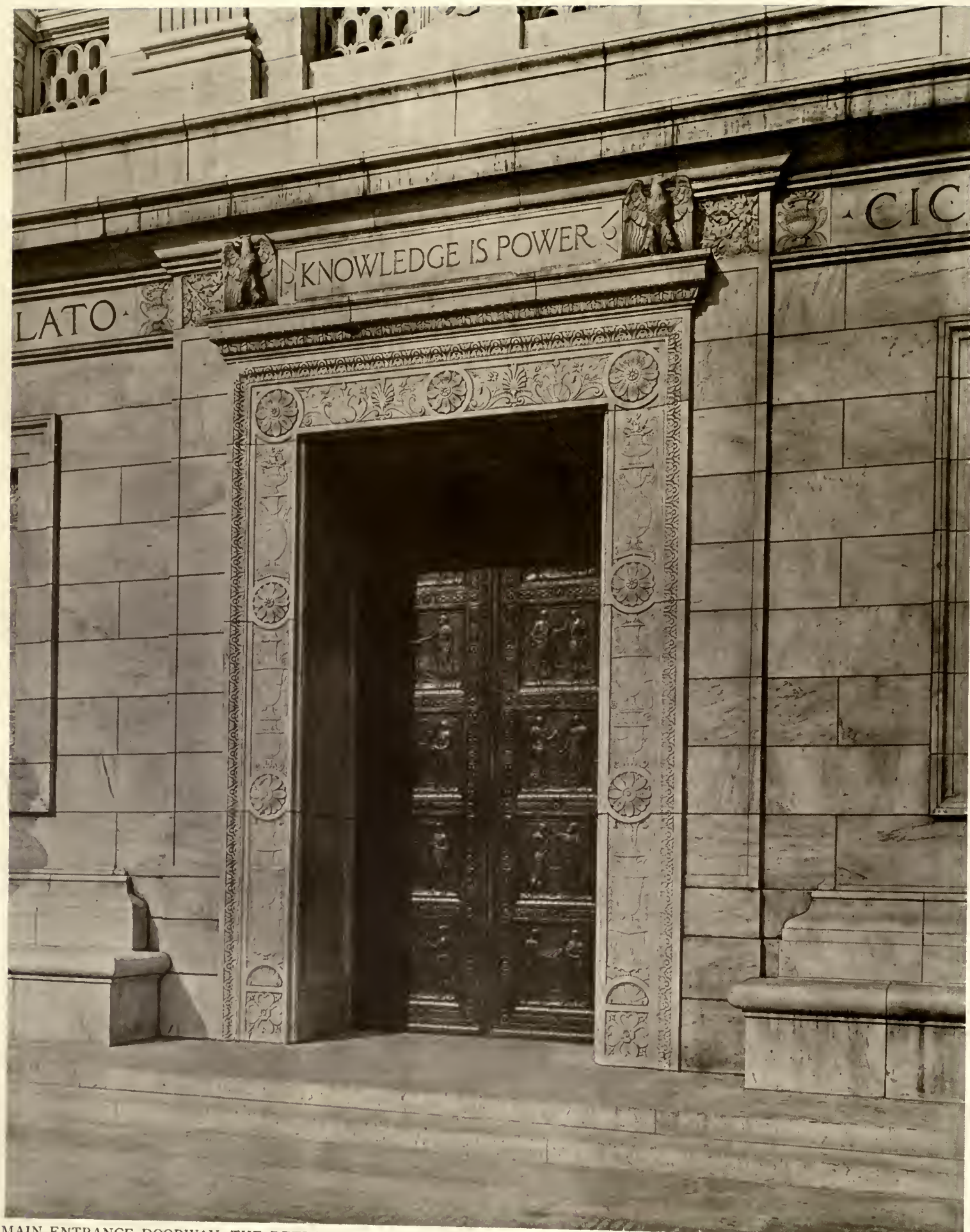
MAIN ENTRANCE-DOORWAY, THE DETROIT PUBLIC LIBRARY, DETROIT, MICH.
