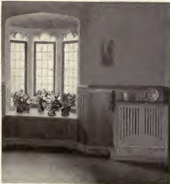
This is a glimpse in the Harkness Memorial. James Gamble Rogers, Architect. A fellow architect, seeing the exposed radiator, suggested this enclosure treatment of wood and Decorative Metal Grille.
