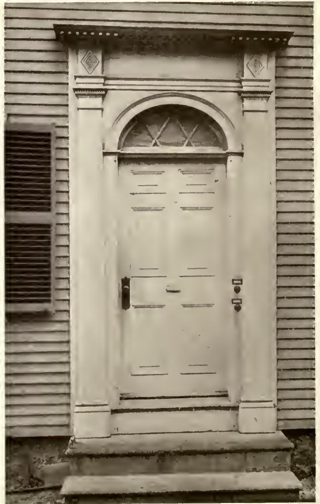
Doorway, Joseph Barnes's house, Plymouth.
