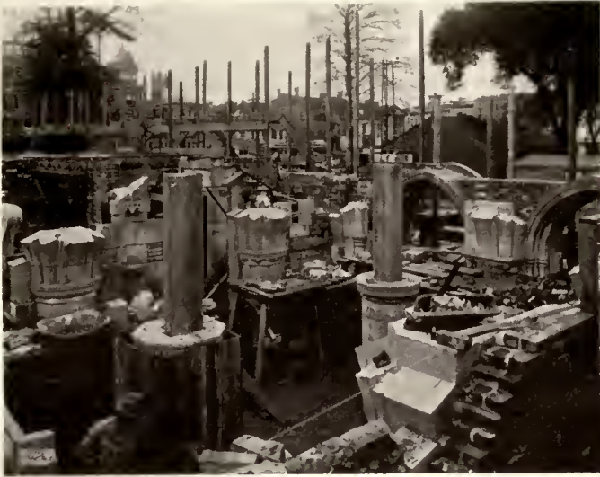
Construction of passage to Calliope Court.
