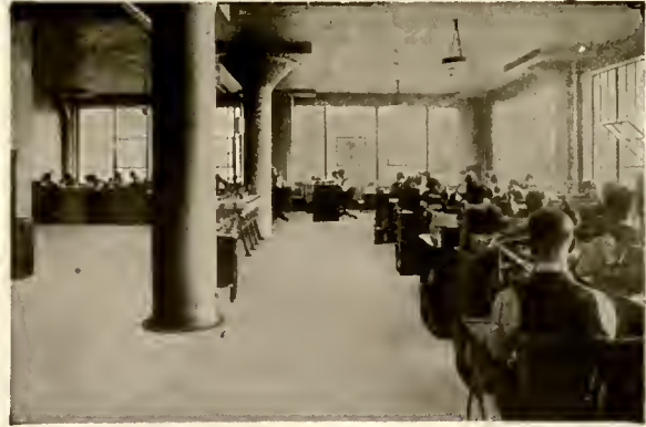
Parker Pen Co., Janesville, Wis. Frank Carpenter, Architect
