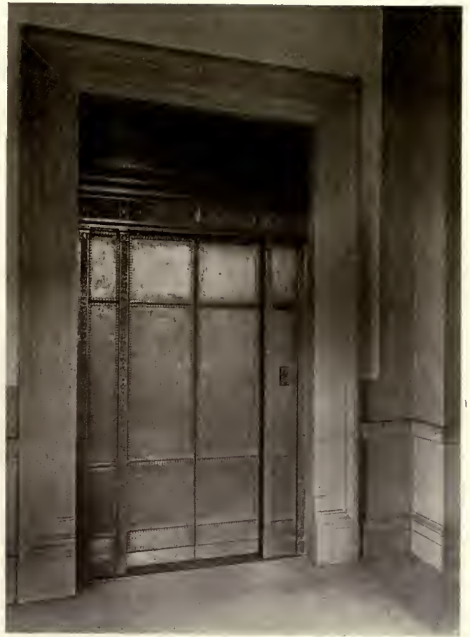
BRONZE ELEVATOR ENCLOSURES.
