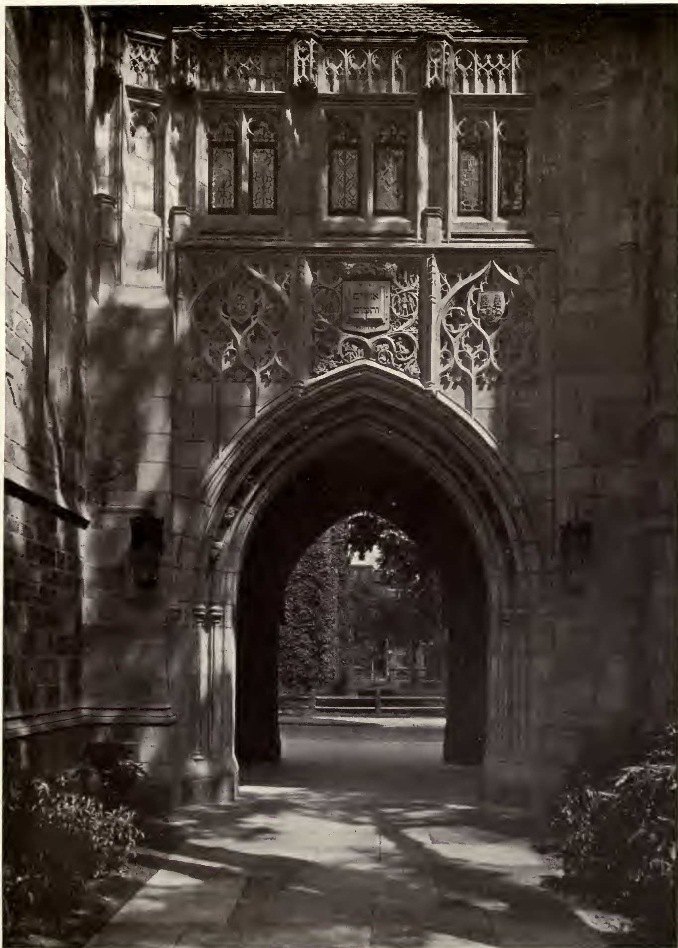
MEMORIAL GATEWAY FROM BRANFORD COURT.
