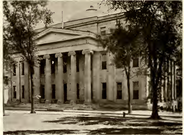
Court of Appeals, State House, Albany, New York. Lewis F. Pilcher, Architect. Windows fabricated by the Tiffany Studios, New York City, from AMBRAC Extruded Bronze shapes manufactured by The American Brass Company.
