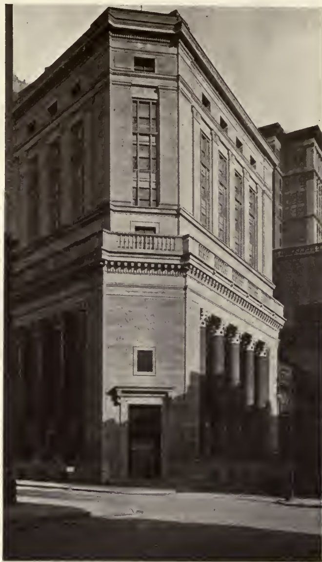
SEABOARD NATIONAL BANK BUILDING, NEW YORK ALFRED C. BOSSOM, Architect Equipped with Sturtevant Apparatus
