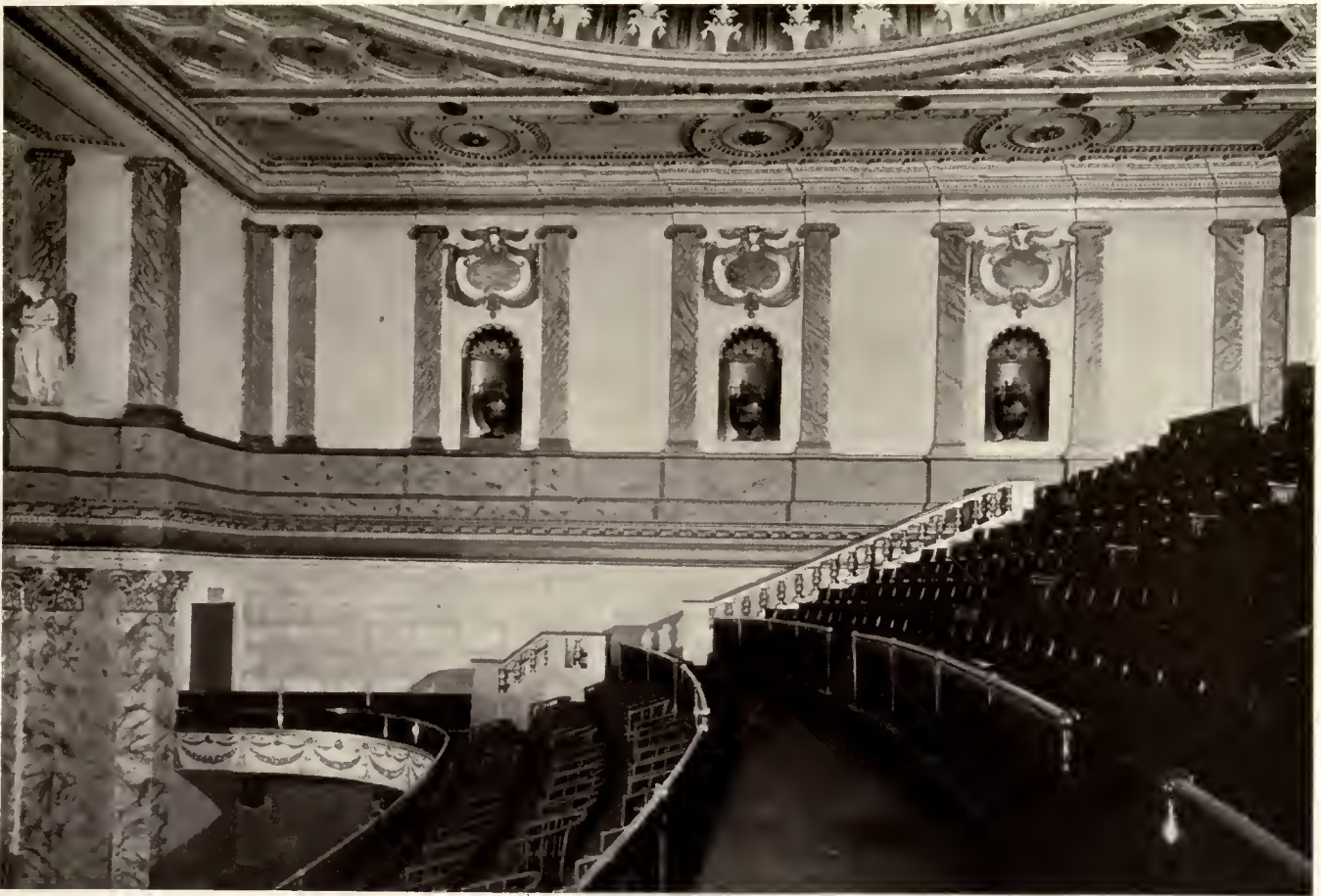
SIDE WALLS OF BALCONY.
