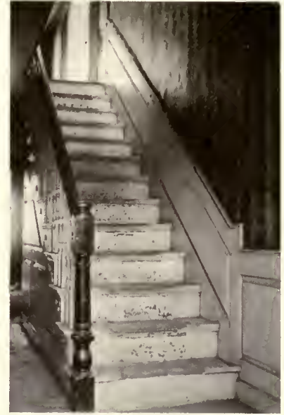
Staircase, Paty house, Plymouth (demolished).
