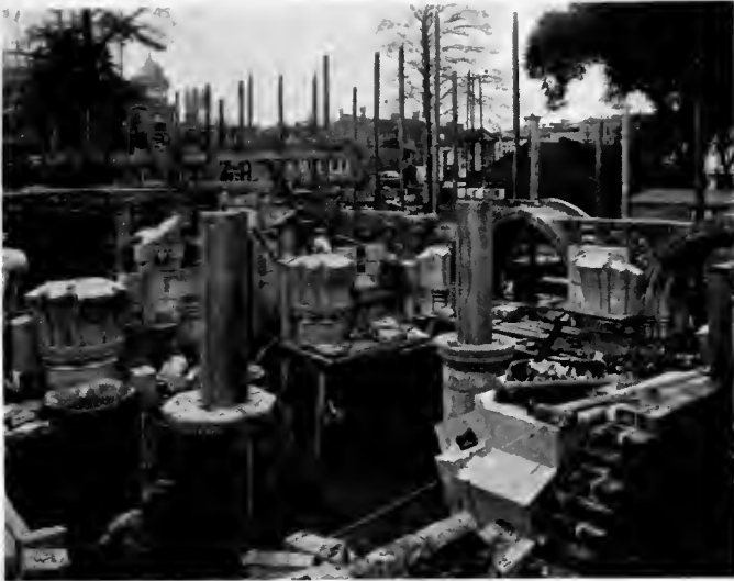
Construction of passage to Calliope Court.
