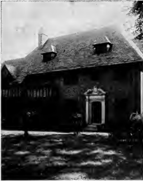
RAPHAEL HUME, ARCHITECT
