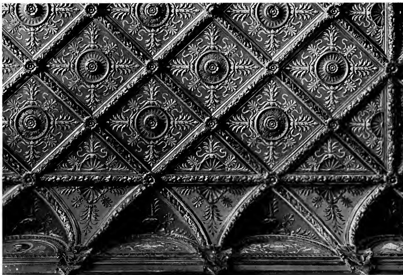
Ornamental plaster ceiling, Social Science and Civics Room.
