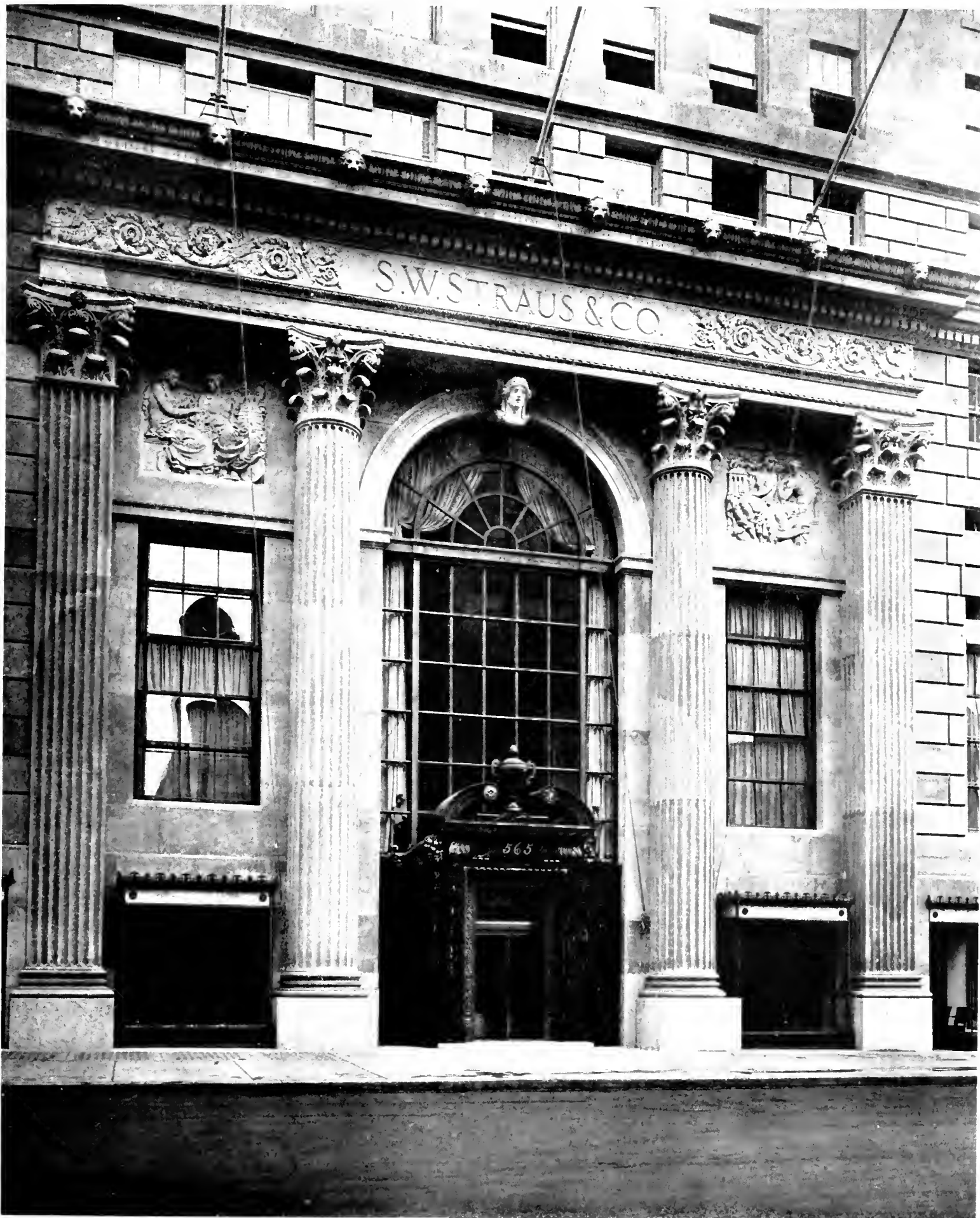
ENTRANCE DETAIL, BANKING HOUSE, S. W. STRAUS & CO., FIFTH AVENUE AND 46th STREET, NEW YORK.
