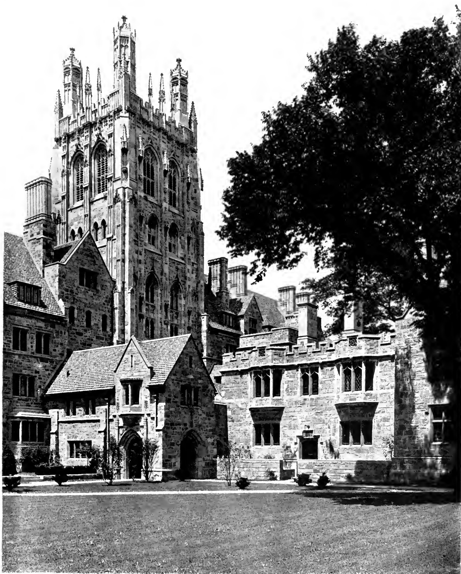
WREXHAM TOWER FROM BRANFORD COURT.
