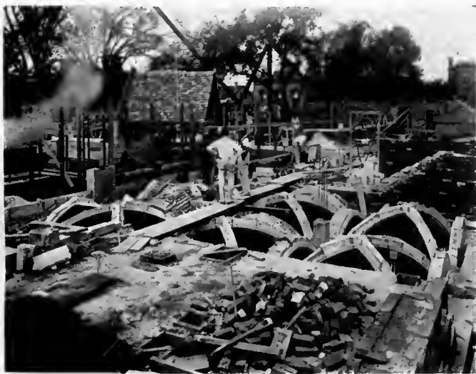
Vaulting of passage to Calliope Court. Sample wall and roof in background.
