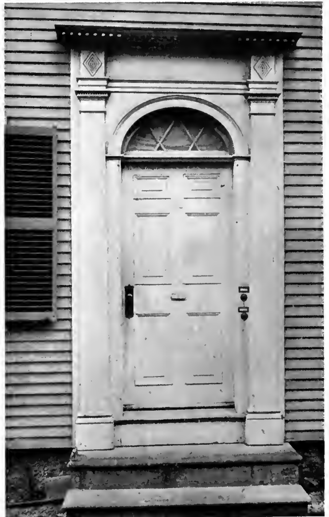
Doorway, Joseph Barnes's house, Plymouth.
