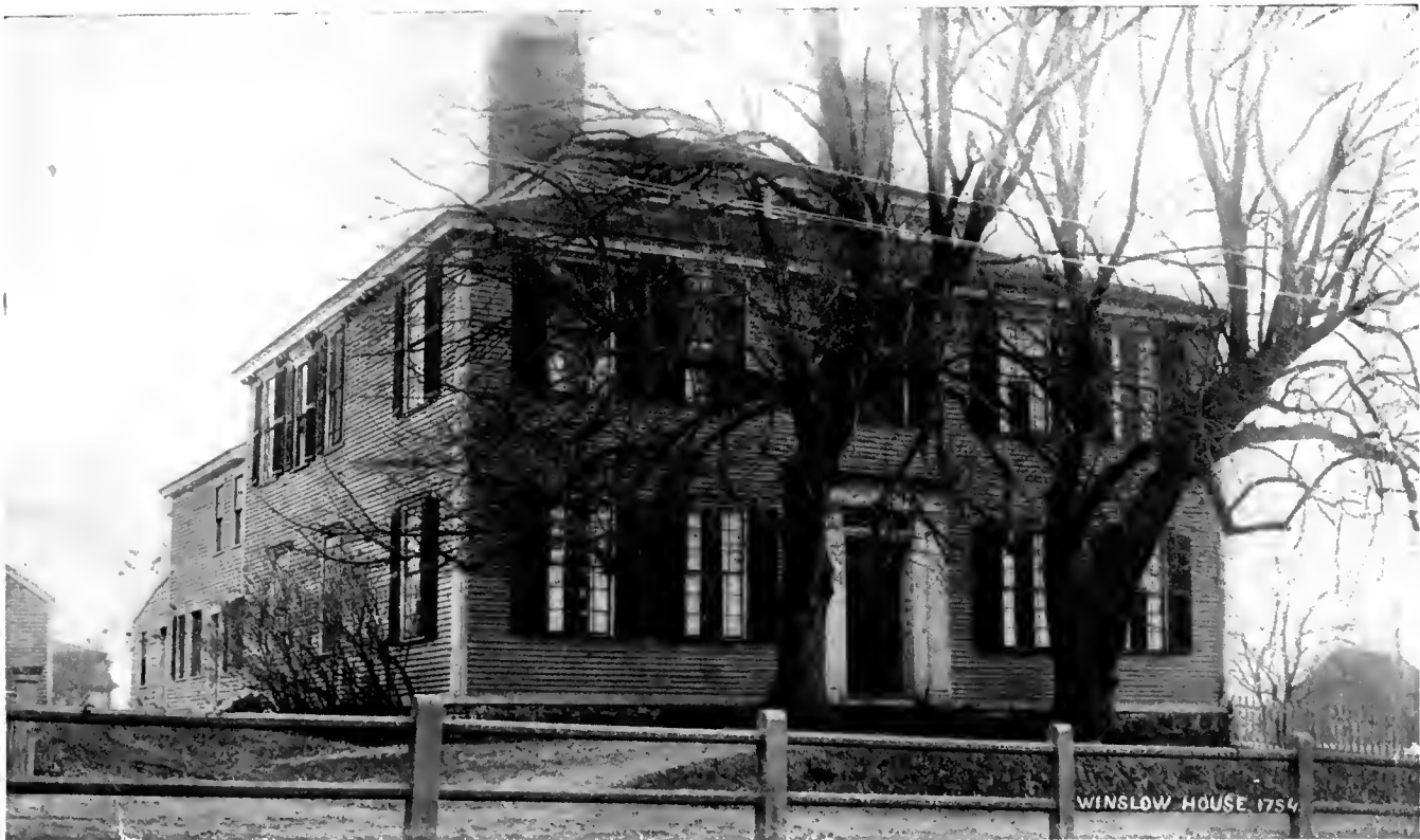
EDWARD WINSLOW HOUSE, NORTH STREET, PLYMOUTH, 1754 (BEFORE ALTERATIONS).
