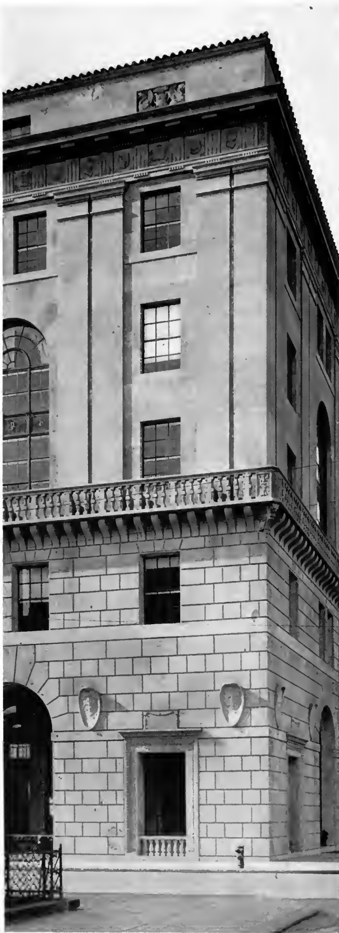
Corner detail, Administration Building, Globe Indemnity Co., Newark, N. J. Frank Goodwillie, Architect. Wesley S. Bessell, Associate.
