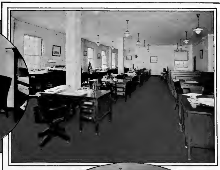
One of the larger offices.
