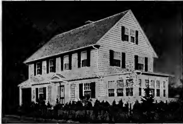
Finished with Cabot's Old Virginia White John Edmund Kelley, Architect, Boston, Mass.
