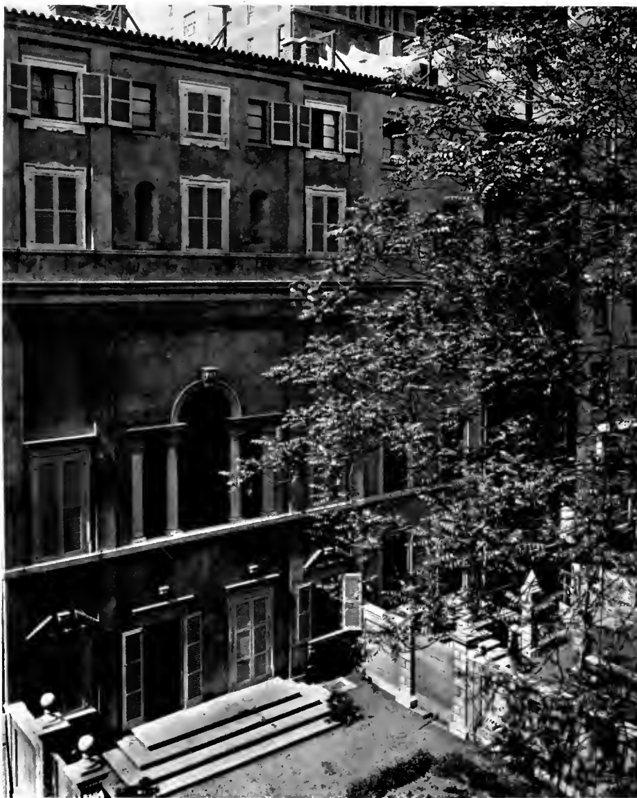
REAR OF HOUSE AND GARDEN.
