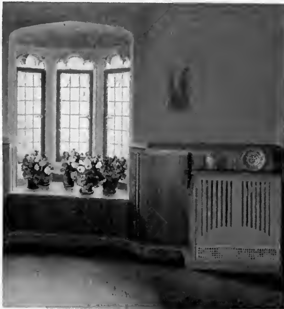
This is a glimpse in the Harkness Memorial. James Gamble Rogers, Architect. A fellow architect, seeing the exposed radiator, suggested this enclosure treatment of wood and Decorative Metal Grille.
