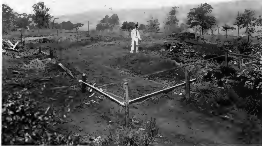
Laying out the work on the ground.
