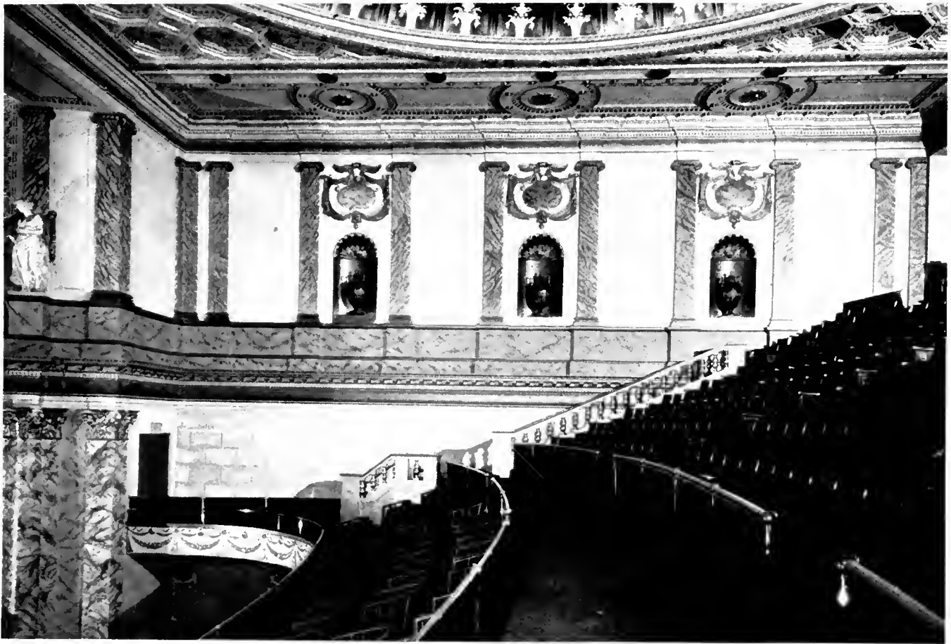
SIDE WALLS OF BALCONY.
