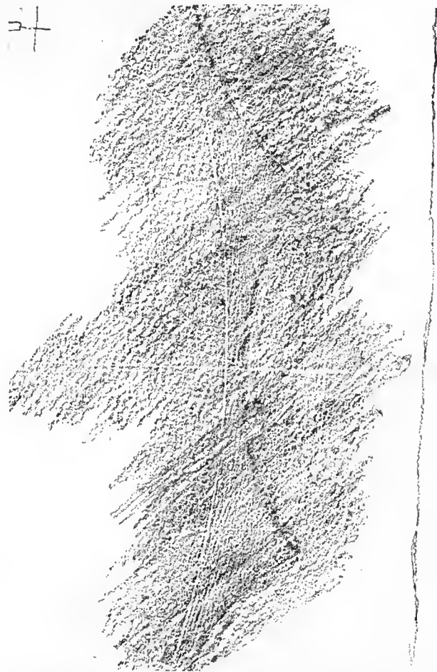
Rubbing direct from base of Tholos, showing methods used by Greek workmen in locating columns. The lines were scratched in the marble. (Rubbing half actual size.)
