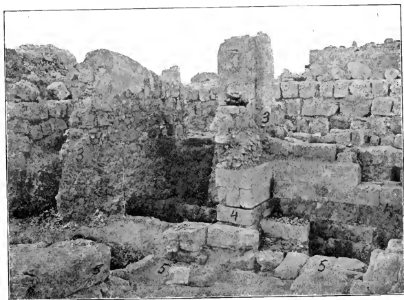
FIG. 42. WALLS OF BUILDINGS AT SAMARIA (after Reisner).
