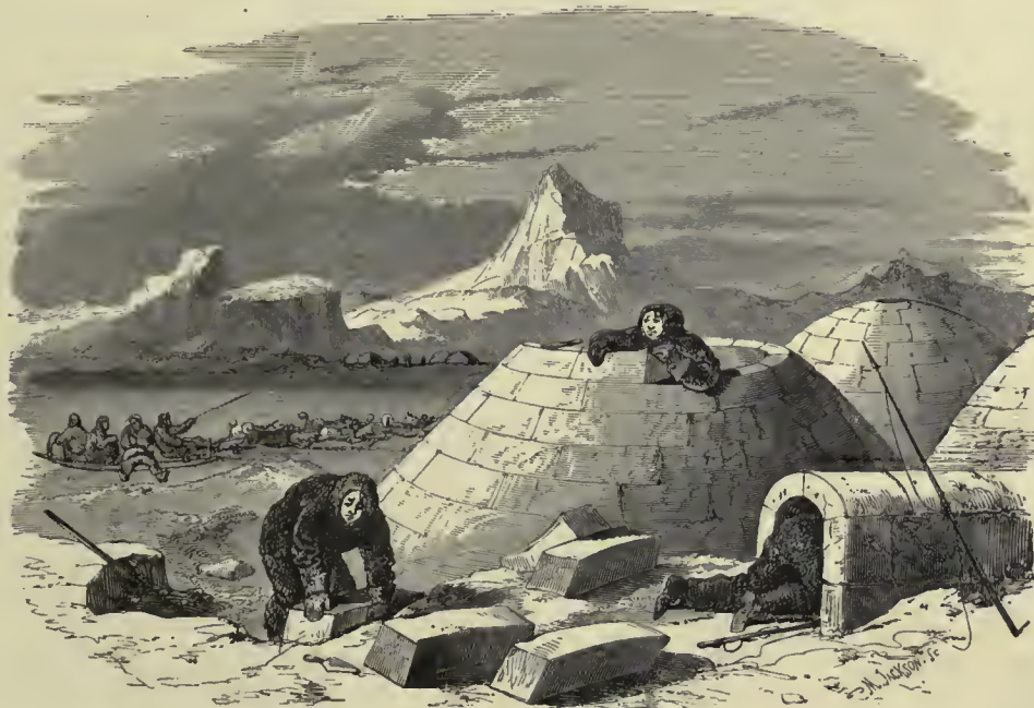
BUILDING AN ESKIMO HUT.
