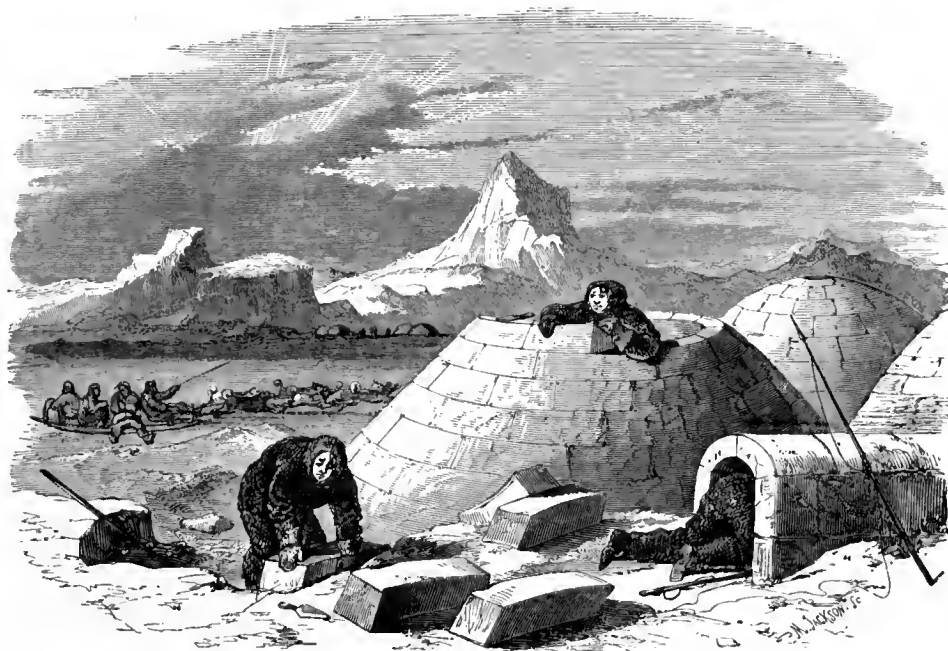
BUILDING AN ESKIMO HUT.
