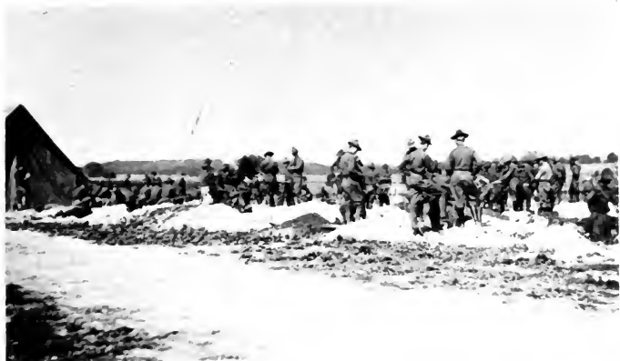
COLLEGE STUDENTS LEARNING THE FINE POINTS OF TRENCH-DIGGING
