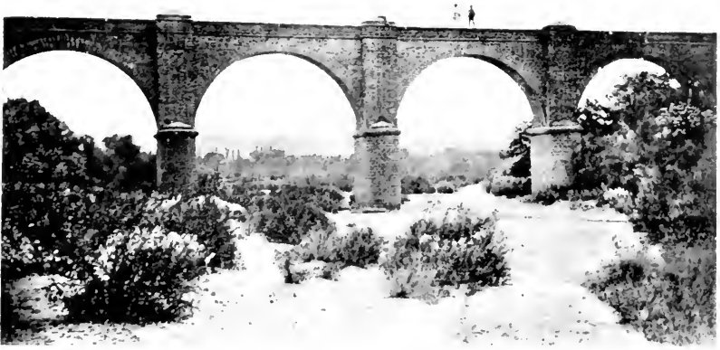
No. 11. AQUEDUCT, SAN LUIS.
