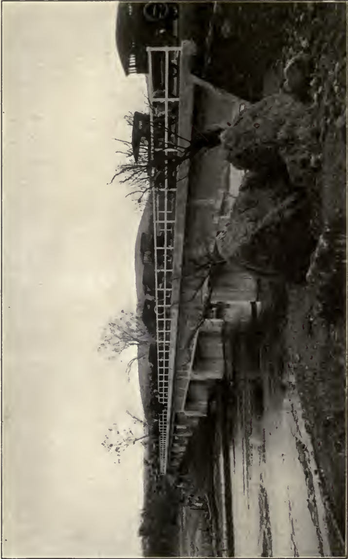
SANTA CRUZ RIVER BRIDGE, NEAR NOGALES, ARIZONA.
