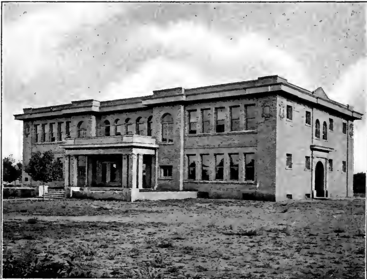
HIGH SCHOOL, DOUGLAS, ARIZONA.
