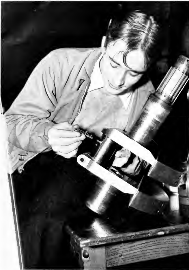
The Guiberson Rotary Diesel has specific application in the United States Army's new high-speed light-weight tank. A student in the engineering defense training program is shown making precise measurements of a Guiberson crankshaft.
