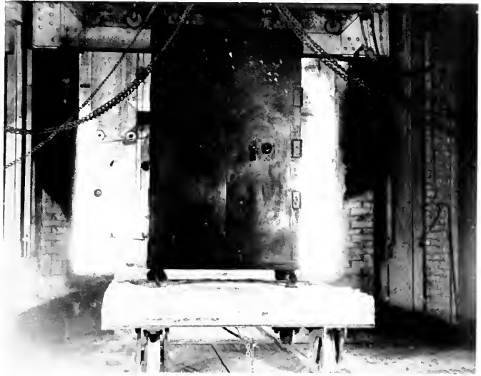
Above: Fire and Load Test of Wall Made of Hollow Concrete Blocks
