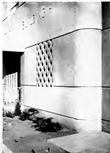
Airport Administration Building, Grand Rapids, Mich., designed for concrete by Spencer Weber, structural engineer, of Lansing. Above close-up shows concrete grilles, rustication and lettering, and fine job of smooth-texture forming. Construction went on during winter months.
