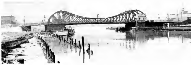
Ninety-Fifth Street Bridge: 1905. 3-Truss, External-Rack Trunnion Bascule.
