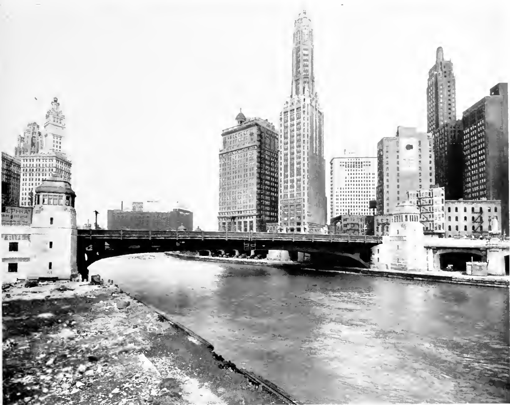
Wabash Avenue Bridge. Trunnion Bascule Type.
