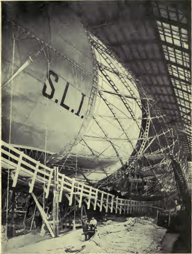
GERMAN AIRSHIP OF THE SCHÜTTE-LANZ TYPE IN COURSE OF CONSTRUCTION.
