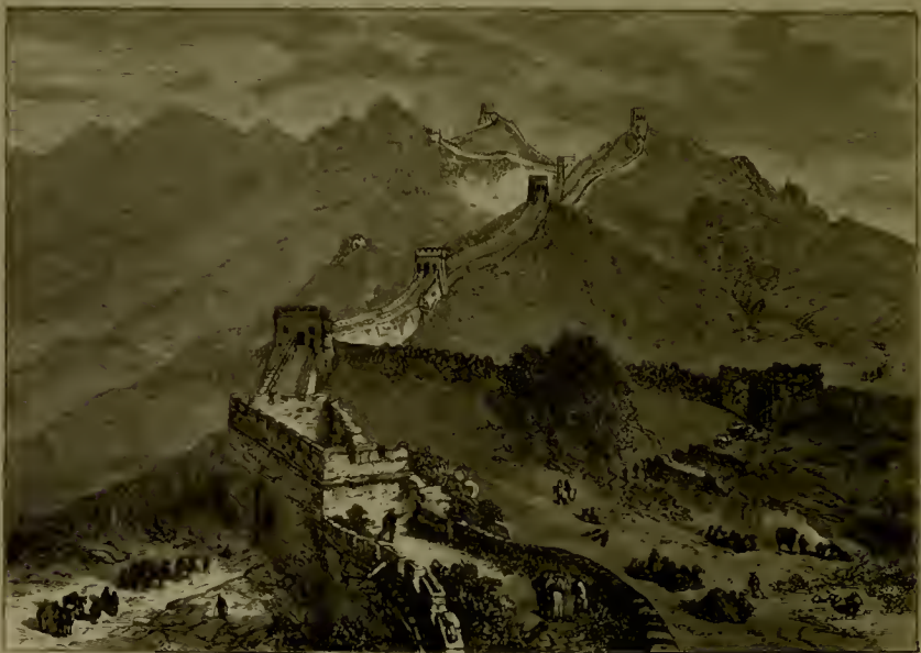
THE GREAT WALL OF CHINA.
