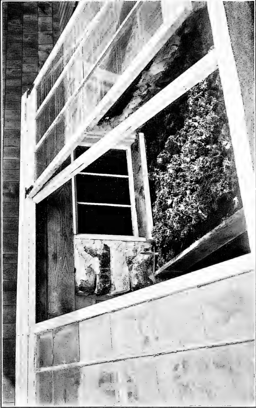
PLATE 23.—Here is a cold frame covered with double glazed sash and heated merely from the furnace room in the cellar, in which lettuce and radishes are grown throughout the winter and plants are started in the spring. Simple, neat, effective.
