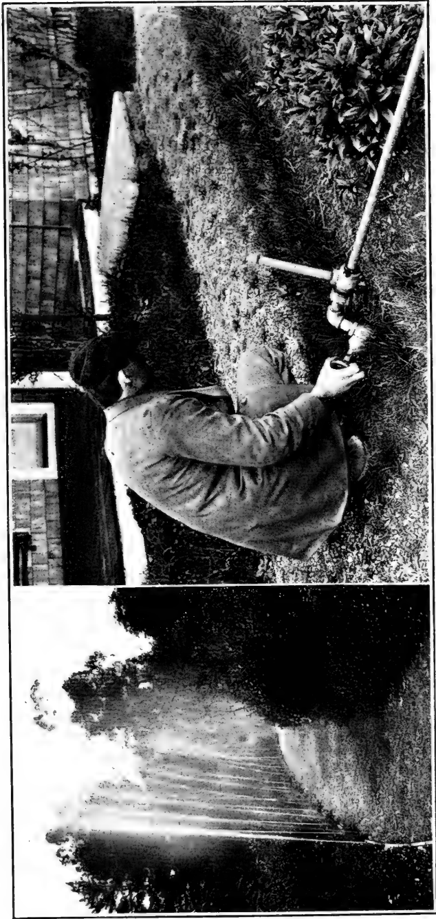
PLATE 14.—(Left) Modern irrigation can be used almost anywhere about the grounds to keep them green and flourishing throughout the summer. When the water is turned off, a line arranged like that in this picture is almost invisible. (Right) This shows the valve by which the water is turned on and off and the special fitting with the strainer and handle by which the line is revolved from one side to the other, adjusting the spray to any position desired over a plot forty to fifty feet wide and as long as the line of pipe. Where wanted, an automatic turning device takes the place of the turning handle.
