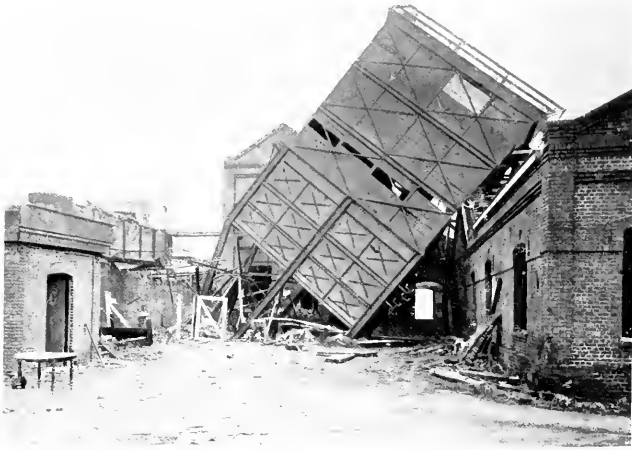
BY-PRODUCT WORKS OF COAL-PITS NOS. 2 AND 2 bis, AT DOURGES, Blown up by the Germans (see p. 114).
