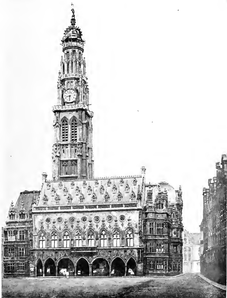
THE HÔTEL DE VILLE AND BELFRY BEFORE THE WAR. The Façade in the Petite Place. Compare with photo, p. 38.
