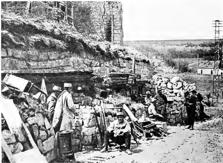
FORTIFIED HOUSES AT THE FOOT OF CARENCY CHURCH, IN MAY 1915.
