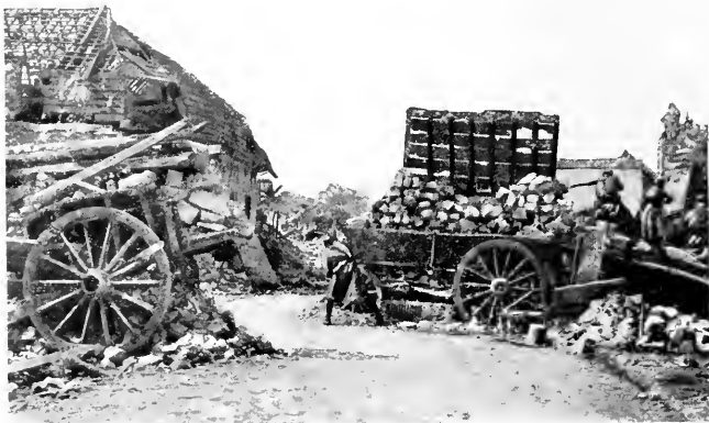
BARRICADE ACROSS THE ROAD AT LA TARGETTE.
