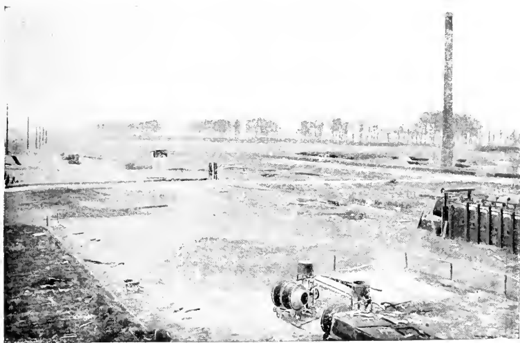
DESTRUCTION OF THE ARBEL WORKS.
