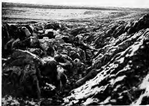
TRENCHES IN FRONT OF SOUCHEZ.
