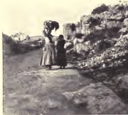
FIG. 8.—The Appian Way of the Republic crossing Monte St. Angelo above Terracina.
