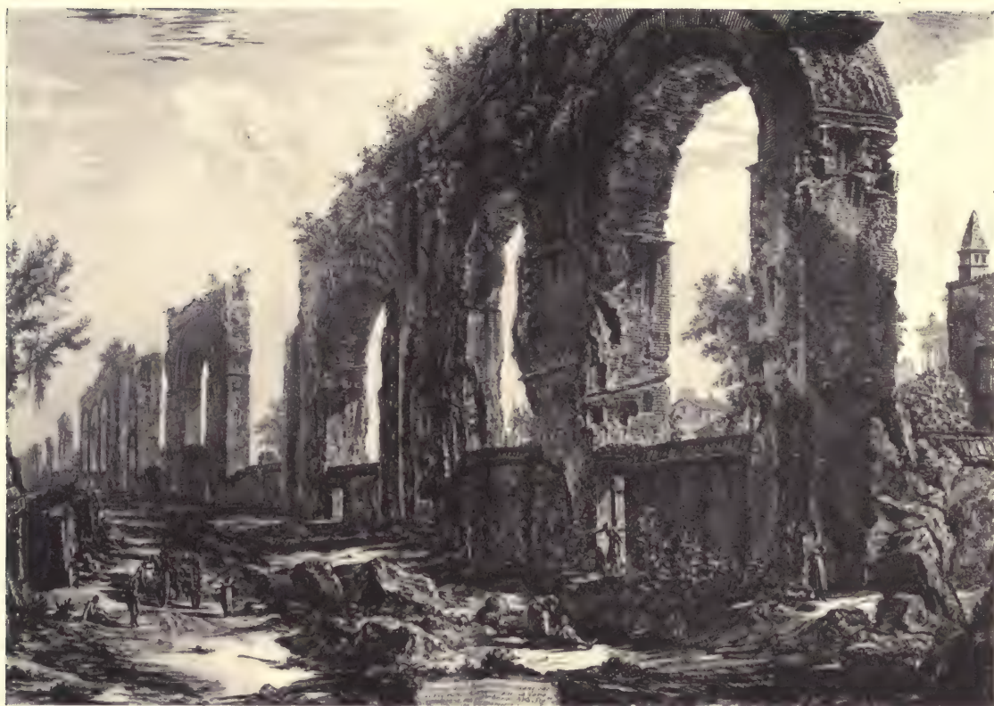
FIG. 5.—Ruins of the Neronian aqueduct, the larger part of which is now inside a private garden in Rome.
