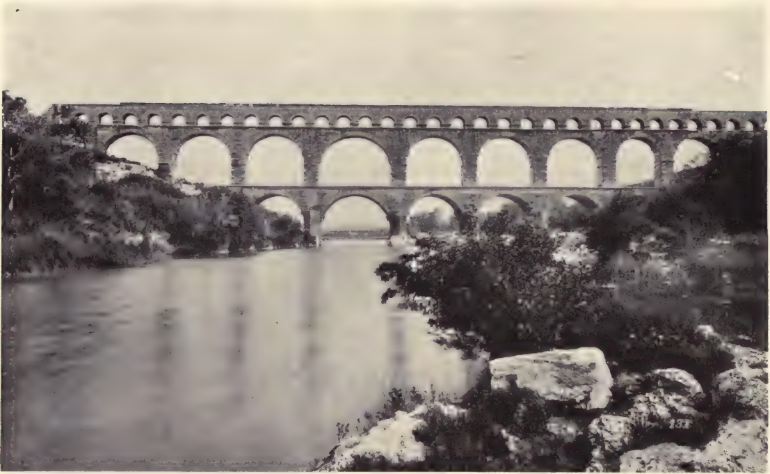
FIG. 5.—The Pont du Gard, near Nîmes.
