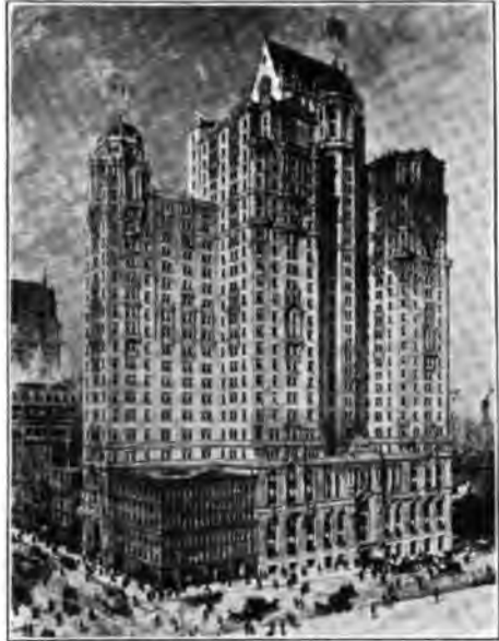
FIG. 87. CITY INVESTING COMPANY BUILDING, BROADWAY, NEAR CORTLAND ST., NEW YORK
