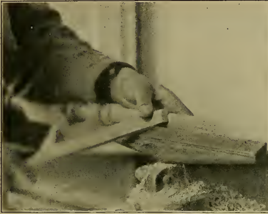
Fig. 58. Turning with One Hand and Supporting the Work with the Other.
