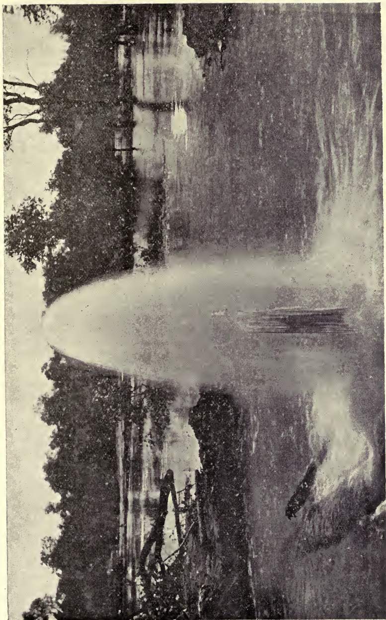
LILA SPRINGS STATION, WARREGO DISTRICT, NEW SOUTH WALES. DEPTH, 1,729 FEET; FLOW, 4,000,000 GALLONS DAILY; TEMP., 124 DEG. FAH.
