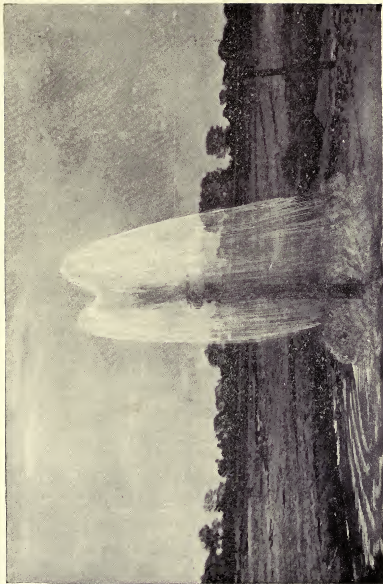
KERRIBREE, BOURKE DISTRICT, NEW SOUTH WALES. DEPTH, 1,340 FEET; FLOW, 1,700,000 GALLONS DAILY; TEMP., 100 DEG. FAH.
