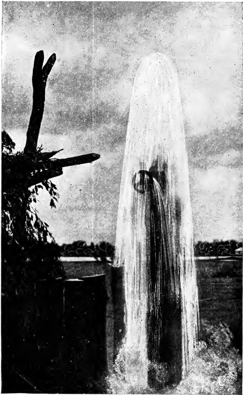
NATIVE DOG, BARRINGUN DISTRICT, NEW SOUTH WALES. DEPTH, 475 FEET ; FLOW, 1,700,000 GALLONS DAILY ; TEMP., 92 DEG. FAH.
