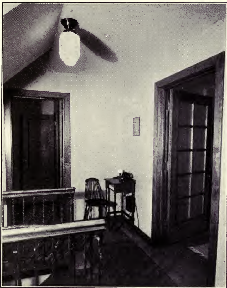
FIG. 24.—This hall fixture with its soft diffusing glassware casts ample light down the stairway. The telephone table is lighted by the midget lamp which also makes a most efficient and inexpensive night light.
