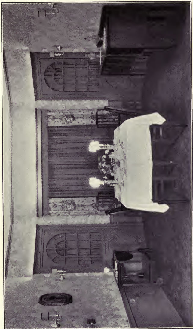
FIG. 35.—The soft light from inconspicuous covers hidden in the window and door frames furnishes a pleasing background for the candlelight dining table.
