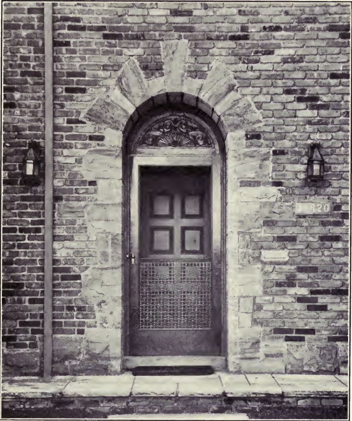
FIG. 23.—The pair of lanterns fulfills the lighting needs of this doorway, and the lighted house number because of its size and position is easily visible from the street 150 feet away.
