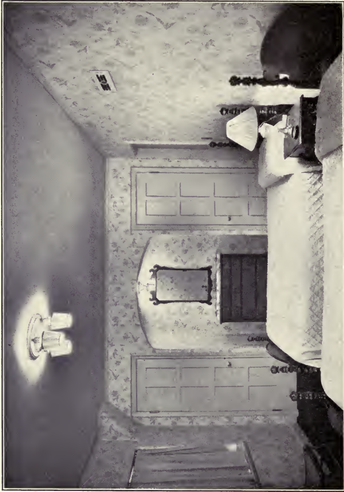
FIG. 38.—The commonplace, uncomfortable, three-light bedroom unit may be made livable by inverted shades. The dresser alcove has its own light (shaded, of course), and the well-designed bed-side table lamp serves both beds equally.
