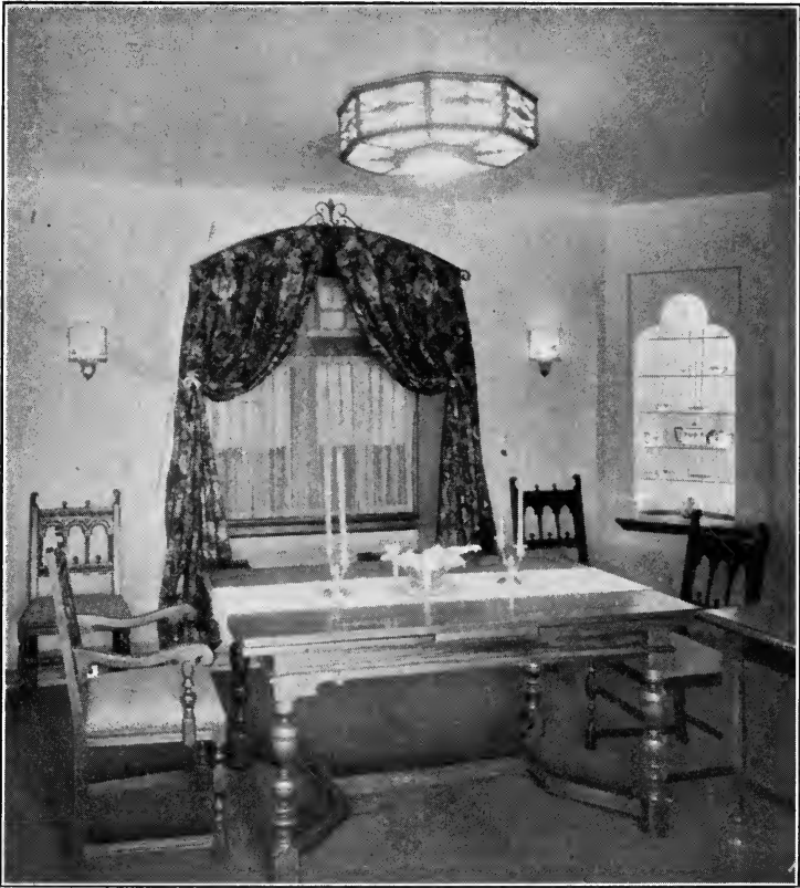
FIG. 36.—This close-to-the-ceiling dining-room fixture has two circuits, one to spotlight the table top and one to lighten the ceiling for general distribution.
