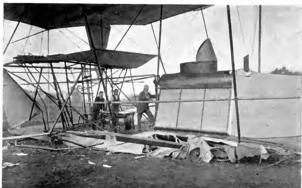
Fig. 82.—The condition of the machine after the accident. One of the broken planks that formed the upper track is shown. It will be observed that the wheels have sunk directly into the ground without leaving any tracks, showing that the machine did not run along the ground, but came directly down when it stopped.
