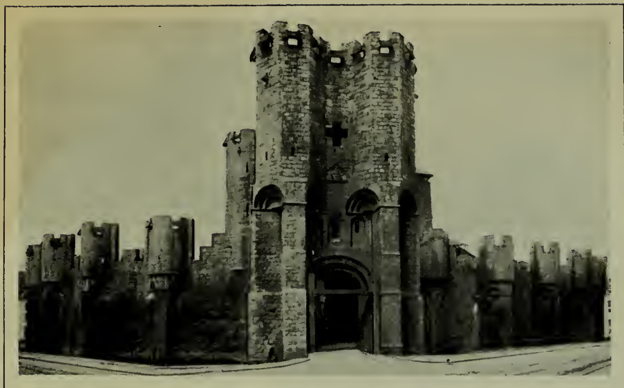
FIG. 1.—GHENT. CHÂTEAU DES COMTES (1180) (General view after recent restoration).
