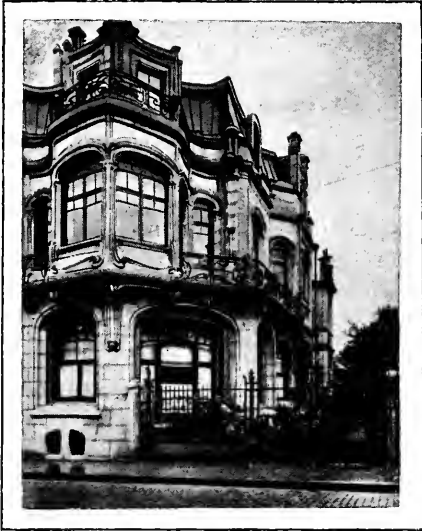
FIG. 536.—VICTOR HORTA. DETAIL OF THE FAÇADE OF THE HÔTEL AUBECQ (550, Avenue Louise, Brussels).
