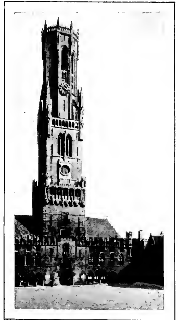
FIG. 41.—BRUGES. BELFRY AND HALL. (Phot. Hermans.)
