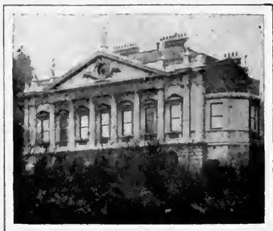
FIG. 199.—SPENCER HOUSE, ST. JAMES'S, LONDON. (VARDY.)
