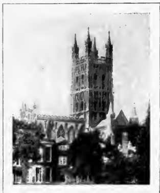
FIG. 137.—CENTRAL TOWER, GLOUCESTER CATHEDRAL.
