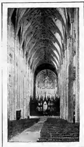
FIG. 108.—WINCHESTER CATHEDRAL, NAVE.
