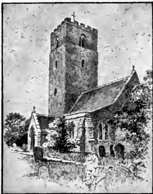
FIG. 34.—CLAPHAM CHURCH, BEDFORDSHIRE.
