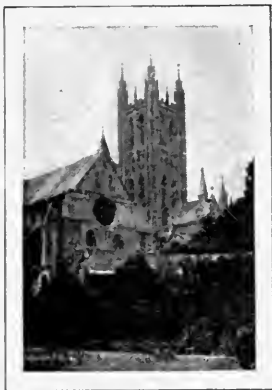
FIG. 91.—ANGEL TOWER, CANTERBURY CATHEDRAL.
