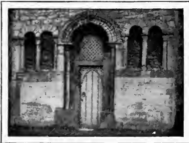
FIG. 33.—BRANSTON CHURCH, LINCOLNSHIRE.
