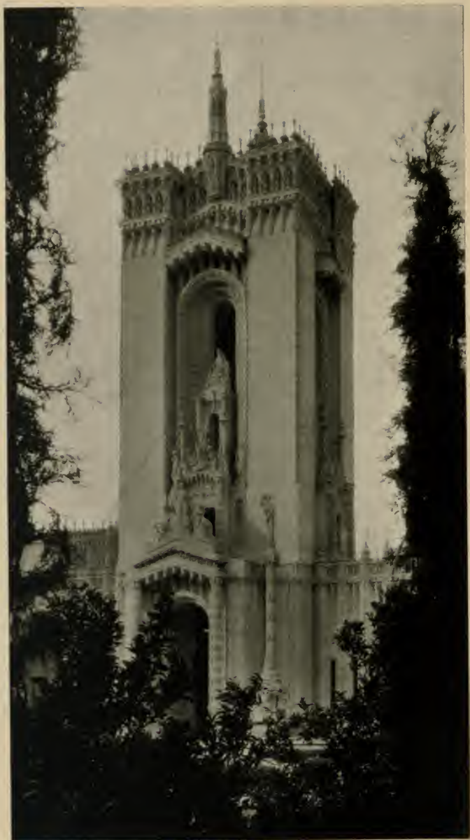
THE TOWER IN THE COURT OF ABUNDANCE LOUIS CHRISTIAN MULLGARDT, ARCHITECT
