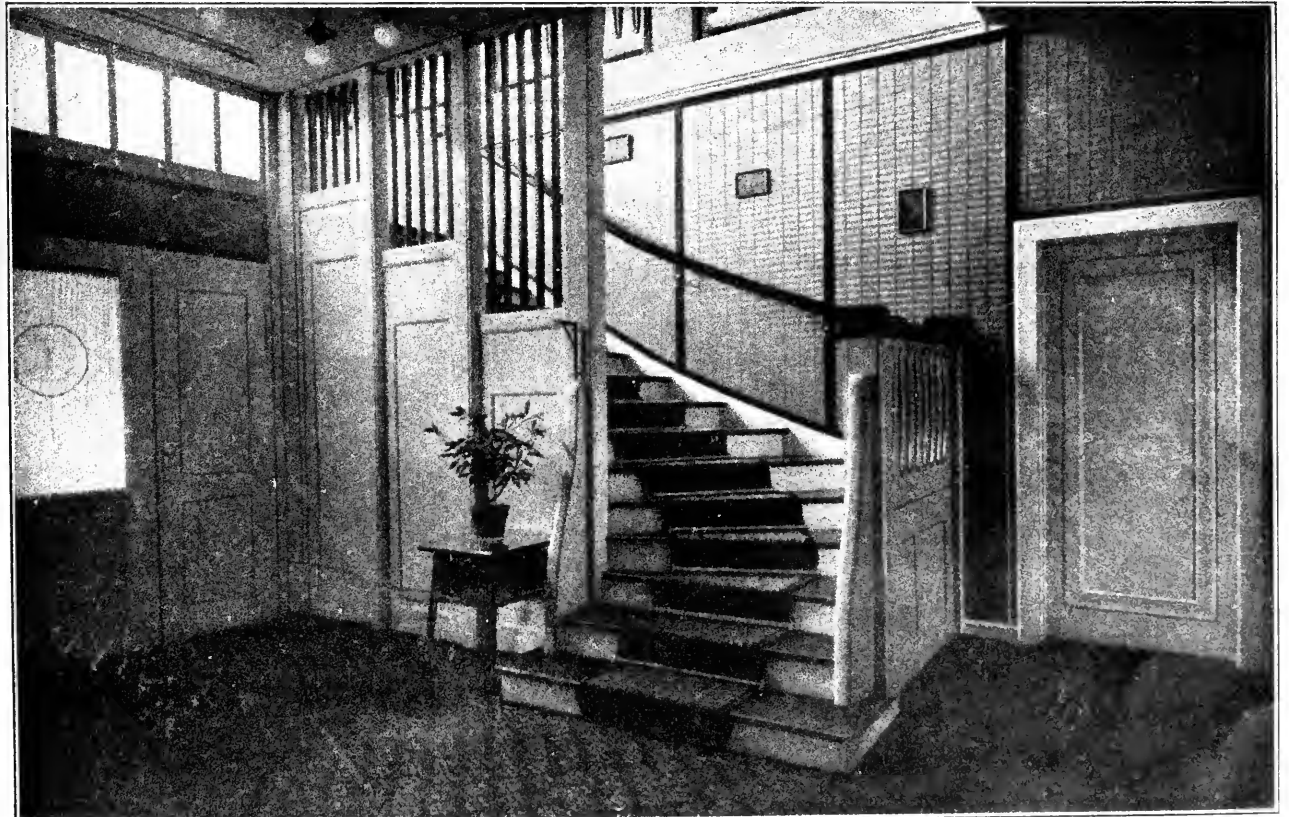
Hall in a European residence, with a quiet, subdued linoleum pattern on the floor
