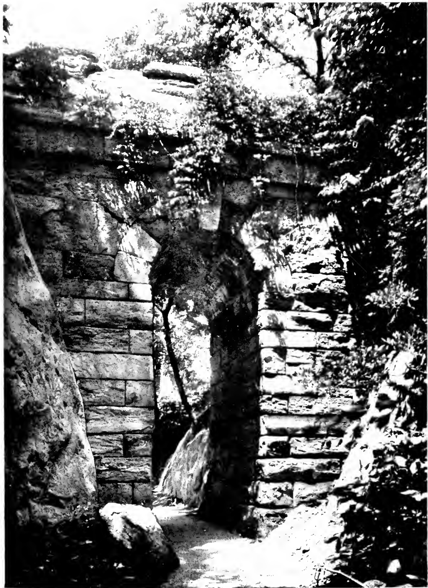
The Rustic Bridge Adjoining the Cave in the Ramble, Central Park, New York City.
