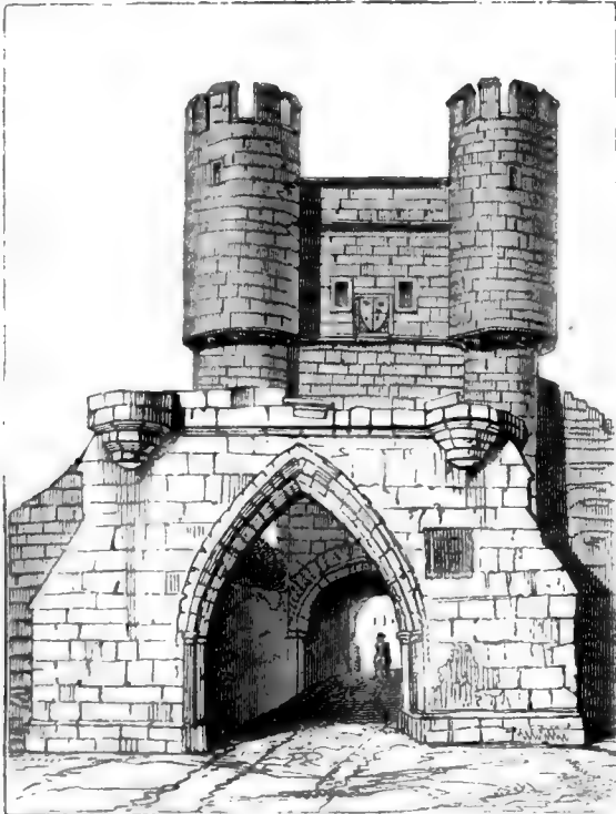
Walmgate Bar and Barbican, York. From "The History and Antiquities of the Fortifications to the City of York," by Messrs. Lockwood and Cates, architects. Lond. 1834.
