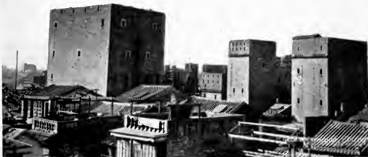
THE PAWNSHOPS OF CANTON These are the only fireproof buildings in the city
