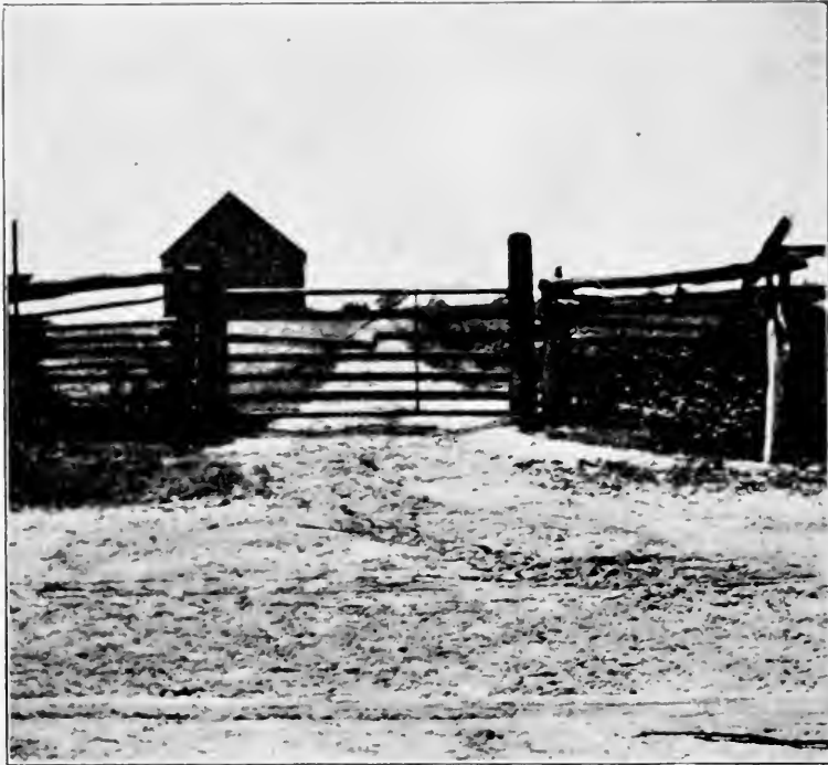
GATE LEADING FROM THE MAIN ROAD TO DR. MUDD'S HOUSE.
