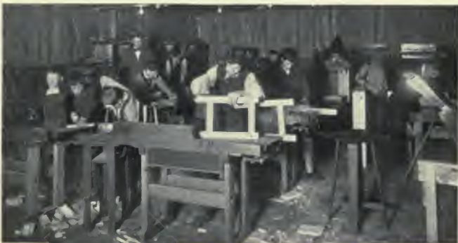
CARPENTRY, BOYS' CLUB—NEW HAVEN, CONN.
