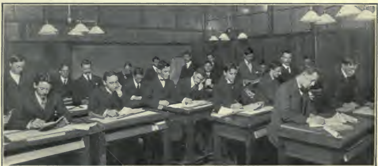
STRUCTURAL ENGINEERING AND DESIGN—WEST SIDE BRANCH, NEW YORK CITY
