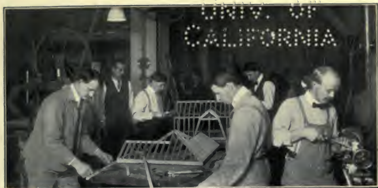
CARPENTRY AND ROOF FRAMING—PORTLAND, ORE.
