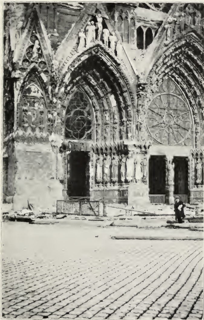
View of damage, main entrance, Rheims Cathedral.
