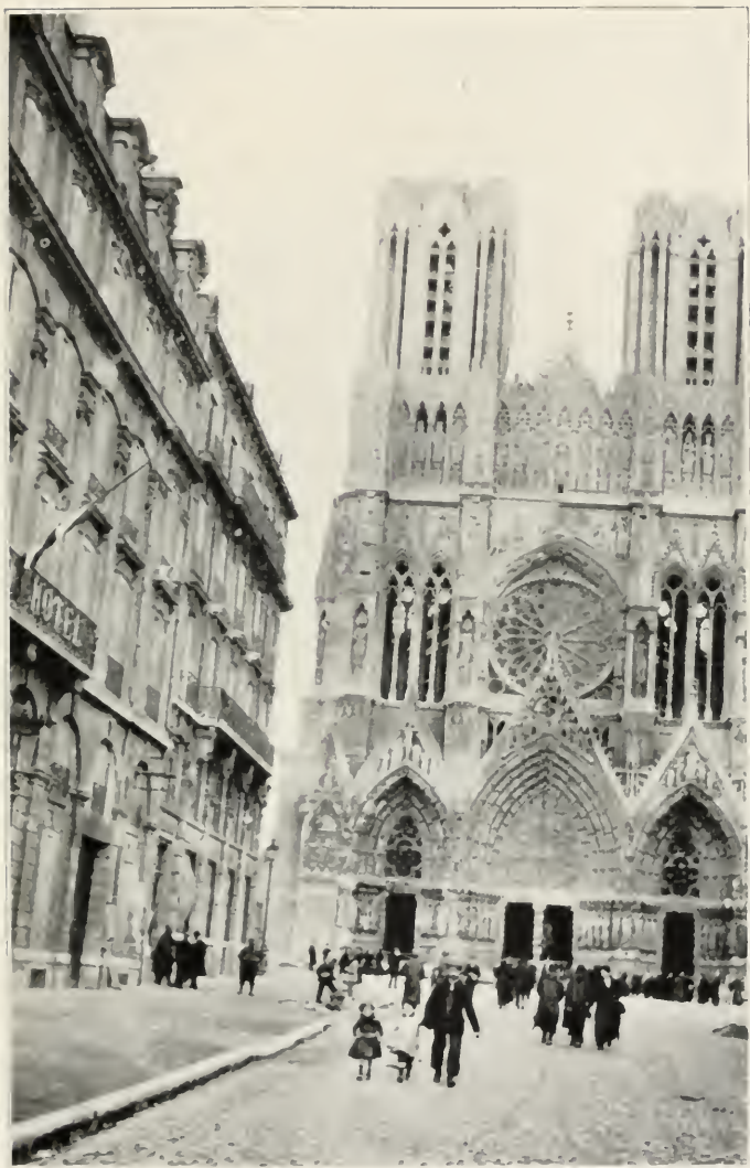
Rheims Cathedral. Notice broken glass windows.
