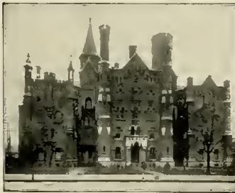
ST. FRANCIS HOSPITAL
