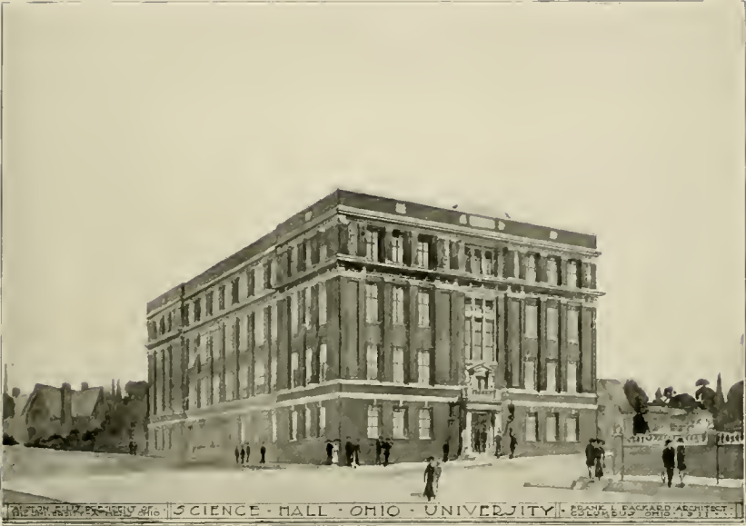
New Science Hall (in process of construction.)
