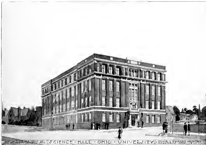
New Science Hall (in process of construction.)
