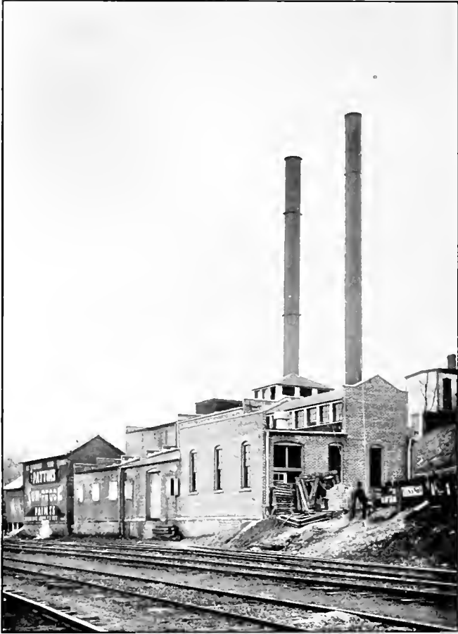
Electric Light and Heating Plant.
