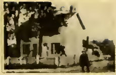
A station on the "Underground" Railroad near Logan about 1865.
