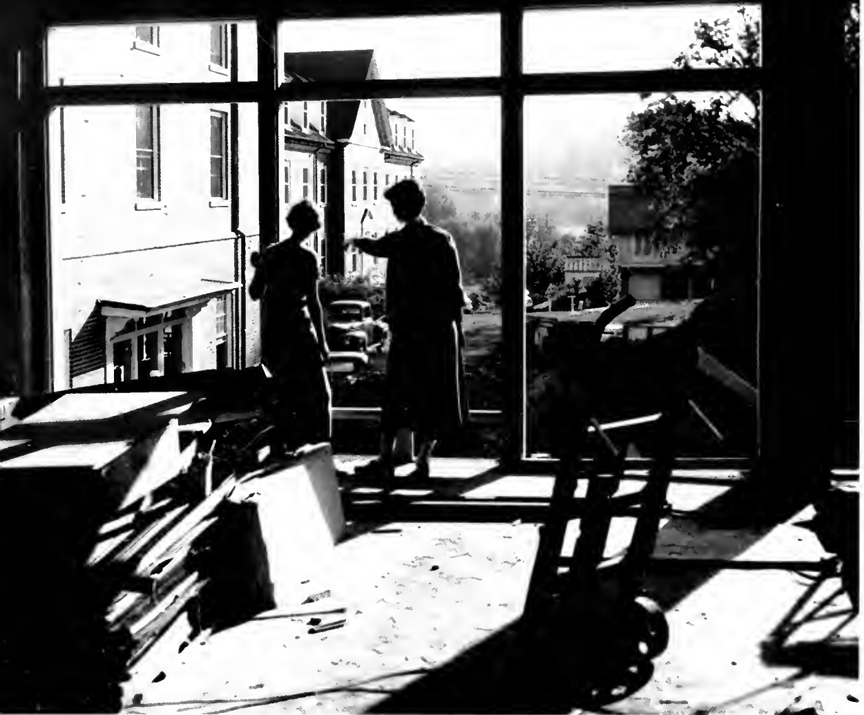
Voigt Hall was still under construction when the girls moved in
