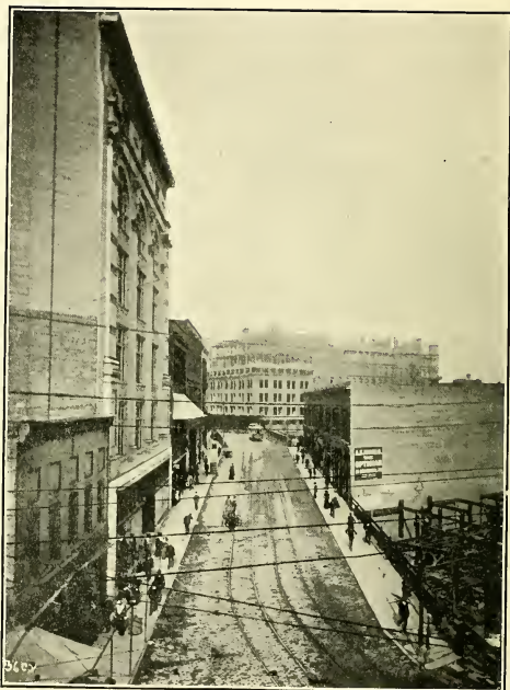
Scene on Whitehall Street Viaduct
