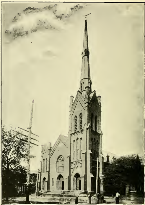
Trinity Methodist Episcopal Church (South)
