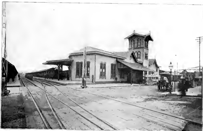
PENNSYLVANIA R. R. TERMINAL, ATLANTIC CITY
