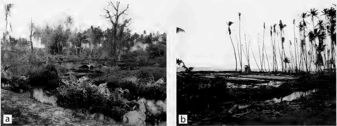
Figure 4. Terrestrial tsunami damage at Pulau Baleh showing (a) dead vegetation along the coast and (b) foundations of buildings that have been washed away by the tsunami wave.
