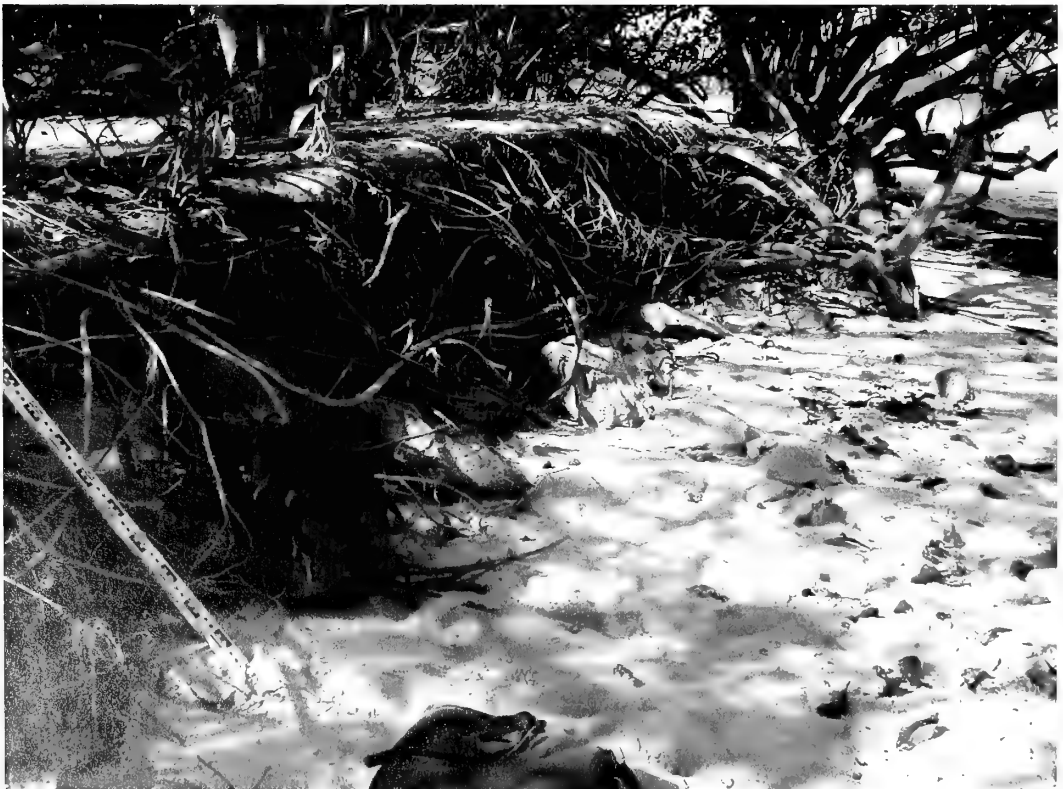
Plate 2. Tsunami-induced scarping and root scour of island margin, northern shoreline of Thilaidhoo.
