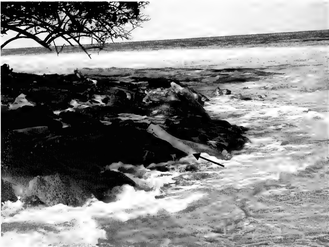
Plate 10. Fractured and imbricated beachrock slabs deposited near the SE point of Hulhudhoo. Slabs to 1.2 x 1.0 x 0.2 m common. Fresh face indicative of fracture and transport during tsunami shown by arrow.
