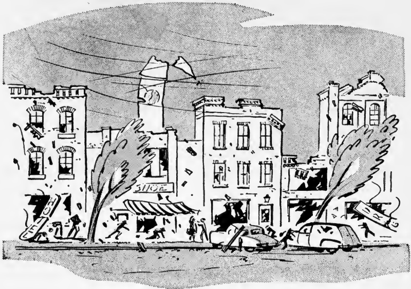
Walls facing the blast may be dished inward—
