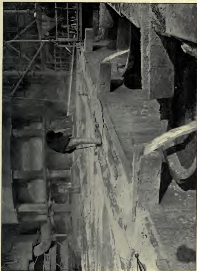
MOLTEN IRON FLOWING INTO "LADLES."
