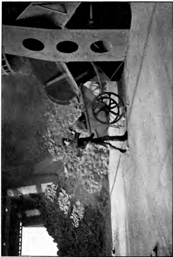
MINE-FILLER DRAWING IRONSTONE FROM KILN.
