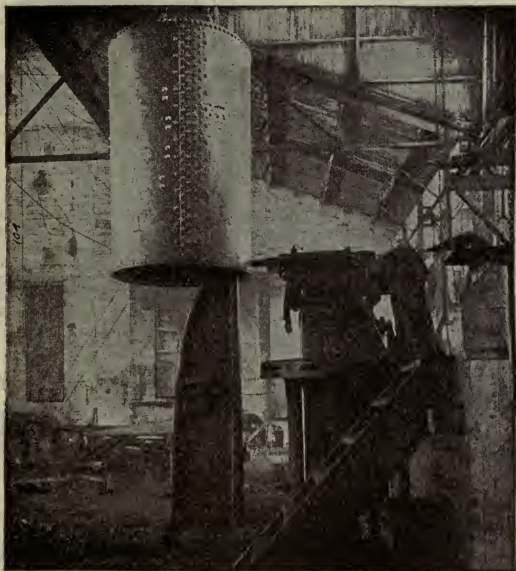
FIG. 4,257.—Hydraulic riveting machine in Freeman & Sons Shop.
