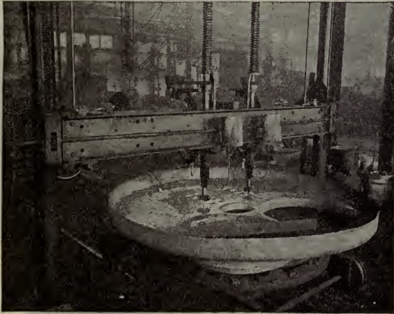
FIG. 4,255.—Multi-tube hole drill. It takes head up to 11\frac{1}{2} feet in diameter.
