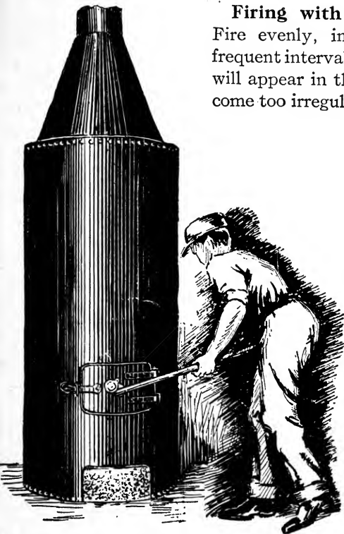
FIG. 4,065.—Firing soft coal in vertical marine boiler of author's steamer "Atlantic City," showing small hole in door, through which slice bar is inserted to break up the fuel. The shutter, loosely pivoted above the hole, falls into place, closing the hole after the bar is removed. This arrangement will be found of great help in firing soft coals.
