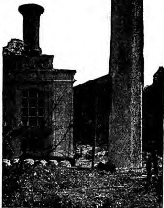
FIG. 4,608.—Heine reinforced concrete chimney in course of construction.
