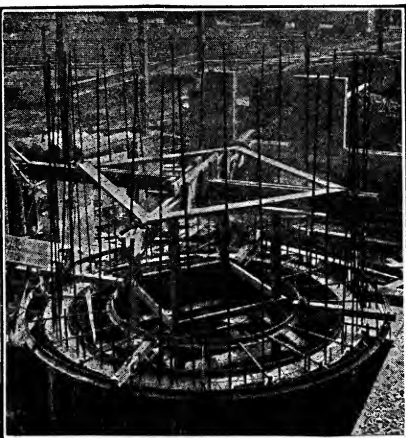
FIG. 4,608.—Heine reinforced concrete chimney in course of construction.
