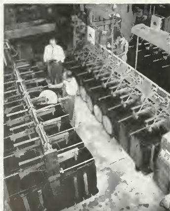
Bank of supplementary copper plating tanks, at the Allied plant. These tank platers are used for non-rush production, increasing the availability of the high-speed plating machines for high priority work.
