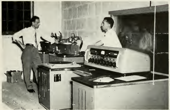
Disc recorders and control console being installed in Protestant Radio Center's headquarters, at Music Building of Agness Scott College, Decatur, Georgia.
