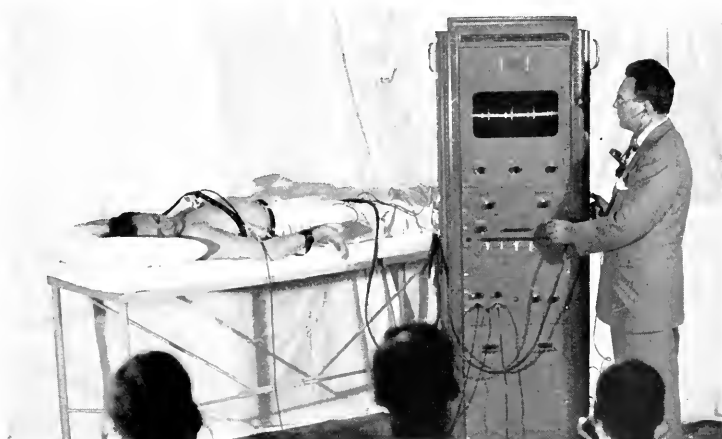
In this typical set-up, the microphone on the patient's chest which feeds into the amplifier in the Educational Cardioscope. The output goes to the individual stethophones of the students and also to the tube of the Cardioscope. The instructor has a microphone and earphones and can talk to the group at will. The tape recorder can be used at the same time for recording the heart sounds.
