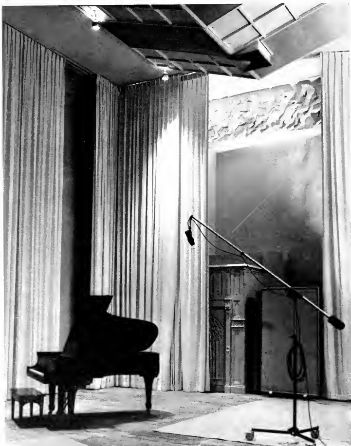
A portion of the main sound studio at Fulton Recording Company, showing the 24-foot high curtains on ceiling tracks which permit variation of acoustical treatment. Studio measures 50 by 35 by 24 feet, closely approaching the theoretically ideal acoustical proportions of 5-3-2.
