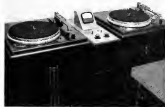
Fig. 2 — Dubbing and playback tables, mounted on special rubber cups and cork sheeting to eliminate building vibration.
